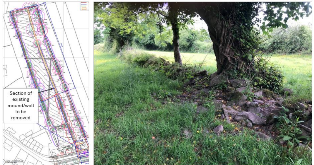
Plate 12 Extract from Demolition Plan showing extent of central wall/mound to be removed hatched in yellow (Left) and Photo showing composition of part of the wall/mound (Right)
